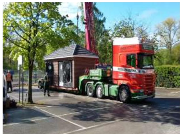
The kiosk arriving by crane
